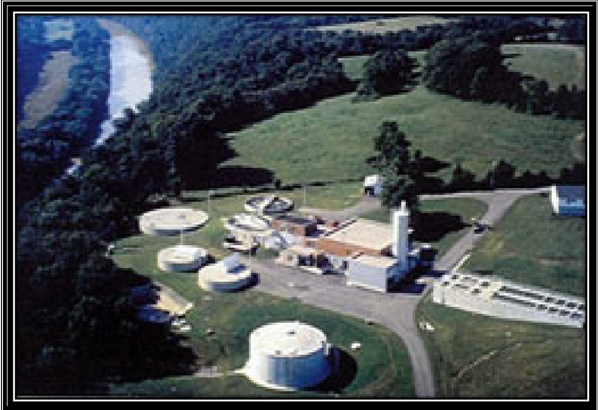
Figure 2 Nicholasville Water Treatment Plant
